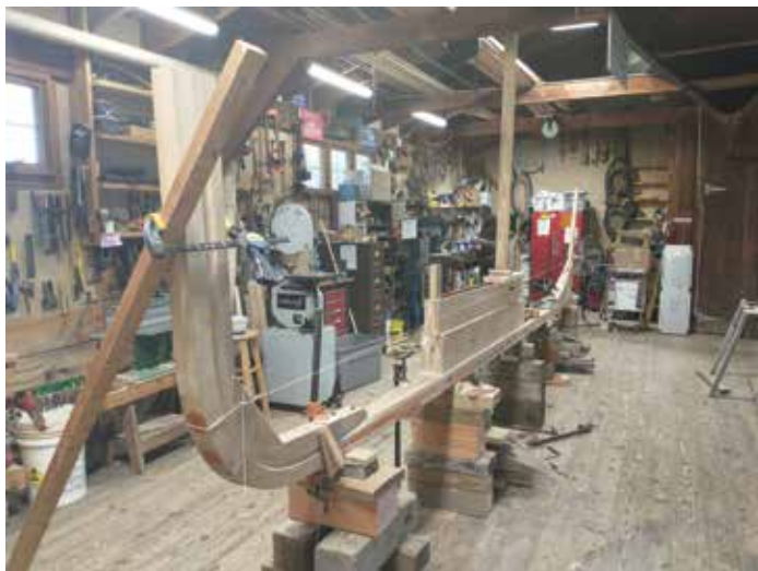
The finished stem, keel, centerboard box, deadwood, and sternpost bedded and bolted in place. The string represents the waterline and this was used to level the boat so that the waterline was parallel to the floor.
