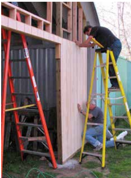
Boat shop endwall construction. (photo by Chris Bickford)
